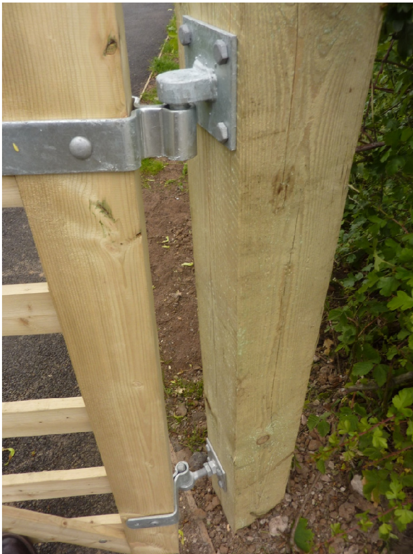
Hinge alignment detail
