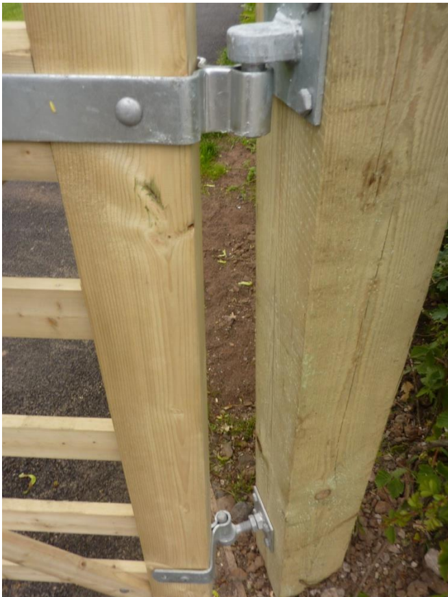
Hinge positioning detail
